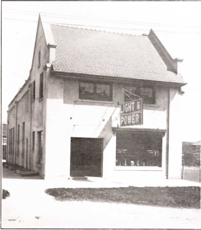
Office and Substation of Eastern Michigan Edison Company
