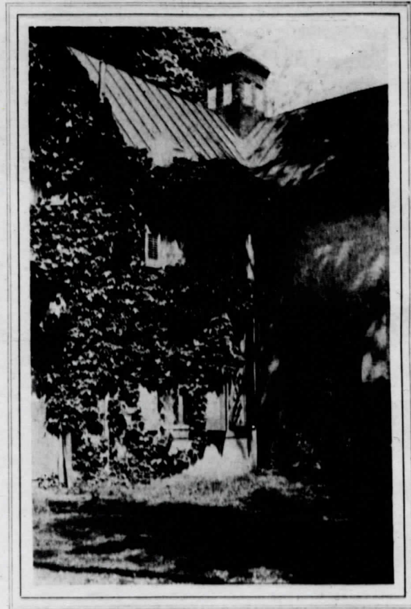
The bay window in the dining-room and, above it, the bedroom window of John Wilkes Booth
