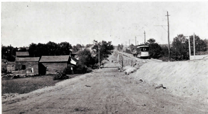
TRESTLE AT ROCHESTER.
