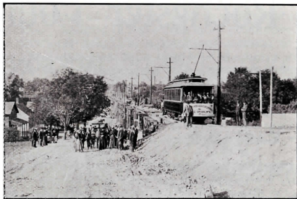
TRESTLE AT ROCHESTER.
